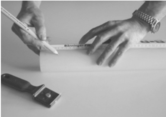
Mark the insertion depth of the sleeve
