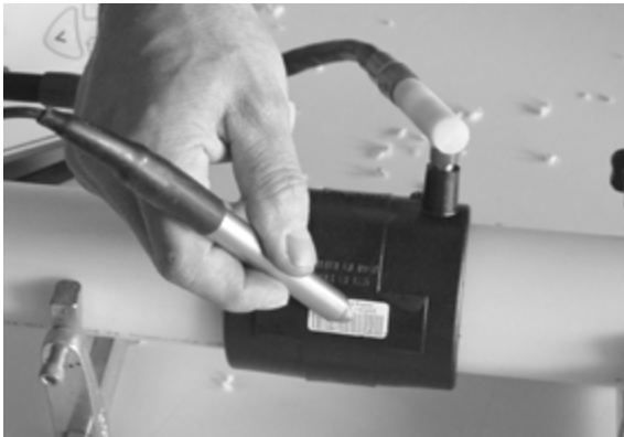
Read in the welding data by scanning the bar code with the bar code reader.
