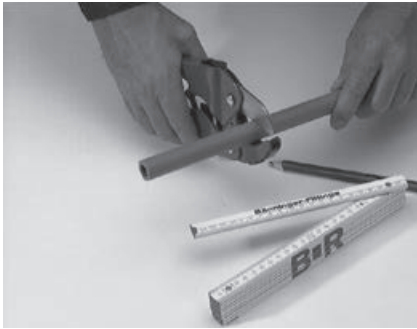
1. Pipes are measured and cut to the required length. Cutting should be rectangular to the pipe axis (90°).
